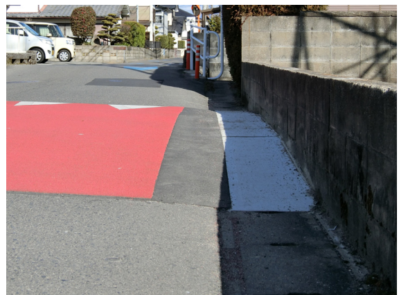
側溝上も併せて嵩上げ
