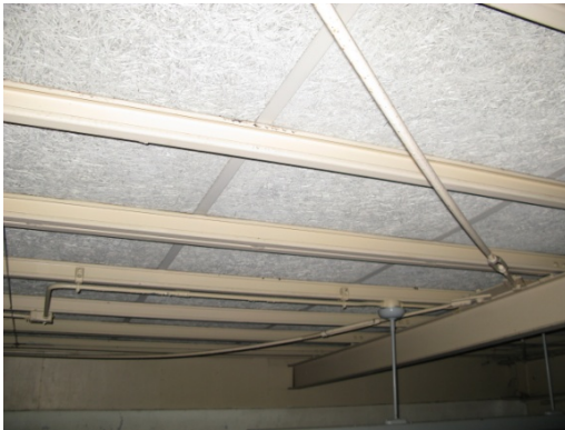
Photo 6.4-9 Deflection of horizontal braces
