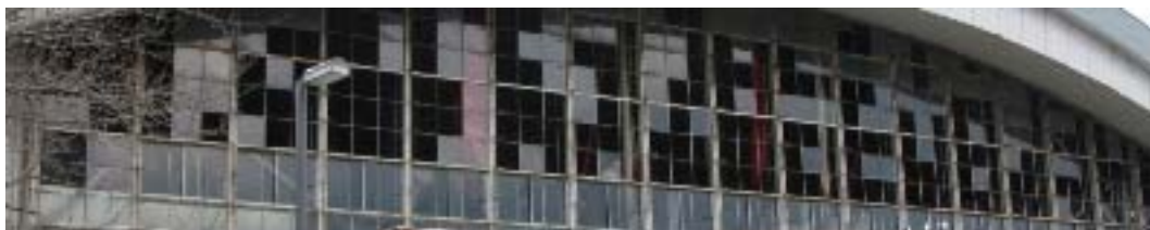
Photo 6.4-19 Breakage of windows
