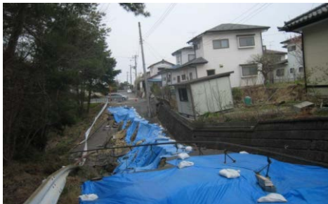
Photo 6.5-17 Fracture of embankment retaining wall and houses tilting by land sliding on the slope of hill end
