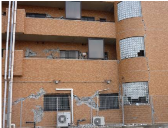
Photo 6.3-43 Damage of nonstructural wall in same building shown in Photo 6.3-22
