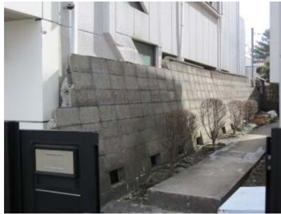
Photo 6.3-51 Collapse of concrete block wall (Sukagawa city)
