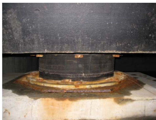
Photo 9.2-10 Rust of High-damping rubber bearing
