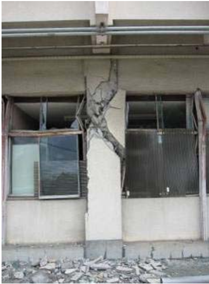
Photo 6.3-18 Shear failure of column
