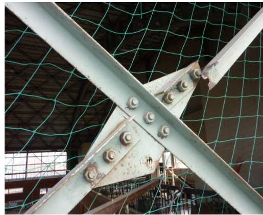
Photo 6.4-2 Net section fracture at bolt hole
