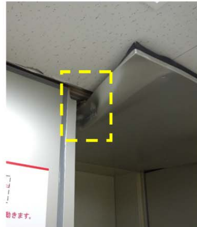
(b) Damage to the expansion joint
