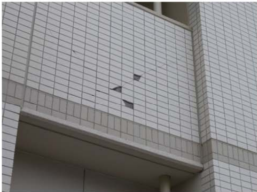
Photo 9.2-13 Drop of ceramic tiles
