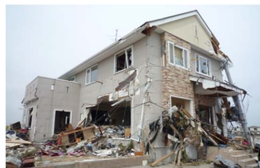
Photo 7.4-19. Light frame construction wood house (12) remained alone
