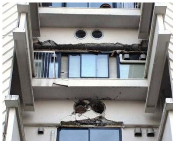
Photo 6.3-28 Damage of boundary beam with opening
