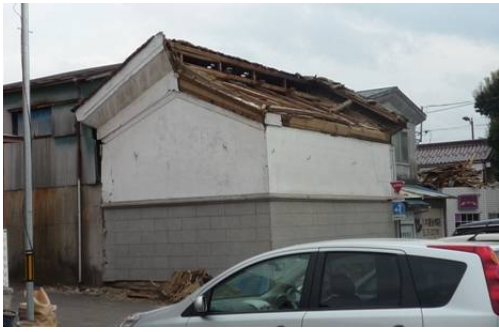
Photo 6.2-48 Fallen roof of warehouse with mud wall
