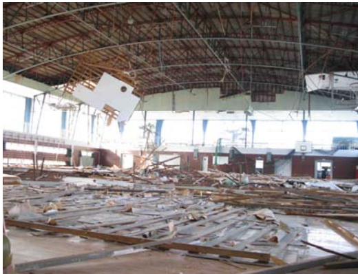
Photo 6.4-16 Dropping of extensive ceiling components
