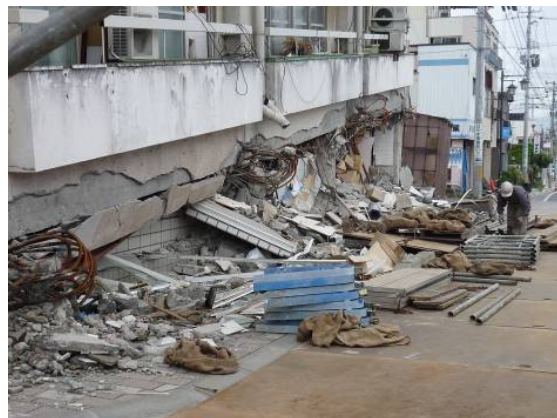
Photo 6.3-3 Close-up view of the fallen story
