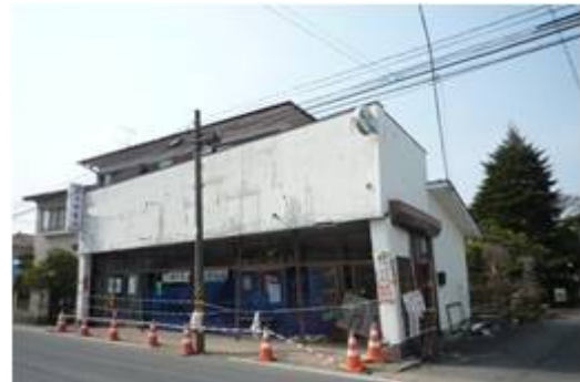
Photo 6.2-20 House with store with large story deformation
