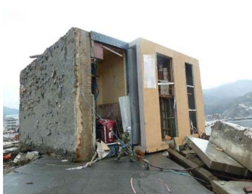
Photo 7.2-2 Overturning of a 3-story reinforced concrete building
