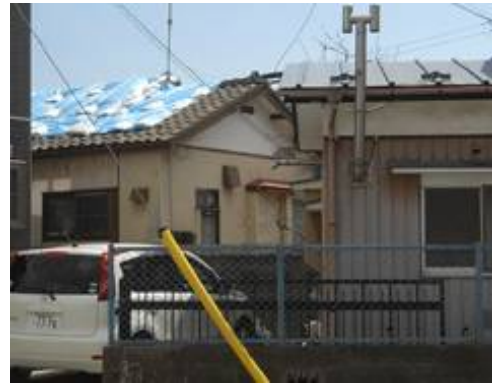
Photo 6.2-34 Damaged roof tile in Hiyorigaoka
