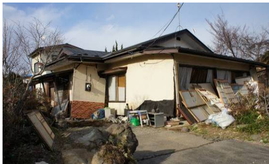
Photo 6.2-63 Wood house with large story drift
