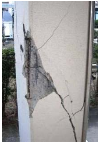
Photo 6.3-13 Shear cracks of first-story columns
