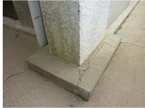
Photo 6.4-12 Cracking of column base concrete
