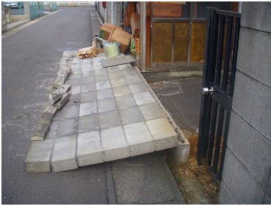
Photo 6.3-50 Collapse of concrete block wall (Koriyama city)
