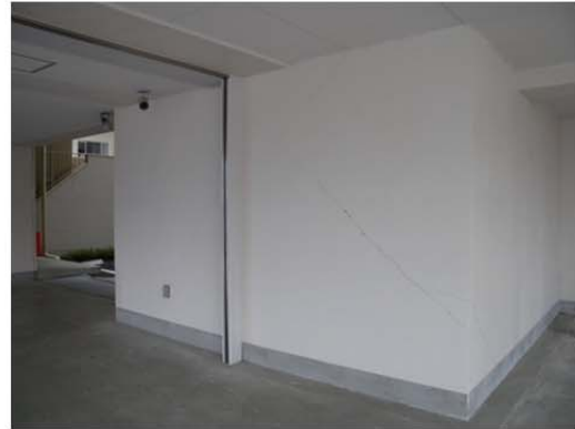
Photo 9.2-14 Shear crack on the wall
