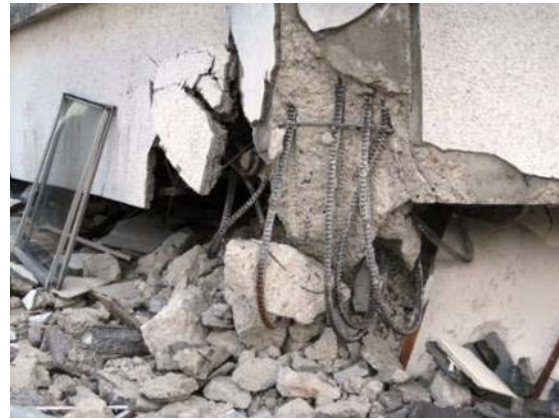
Photo 6.3-5 Close-up view of the fallen story
