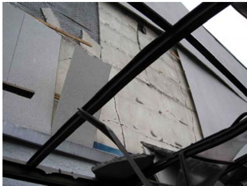
Photo 6.4-20 Falling of exterior finish components
