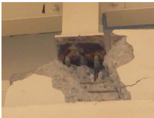
Photo 6.4-6 Spalling of concrete
