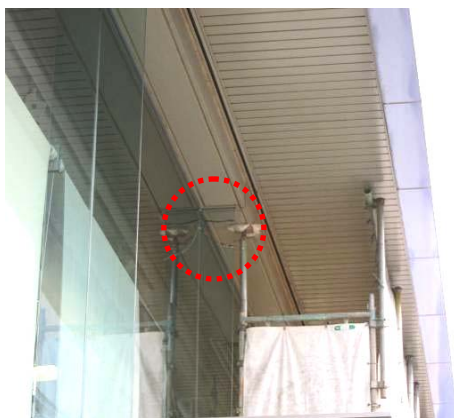
Photo 6.6-12 Breakage of glass mullion of glass wall system
