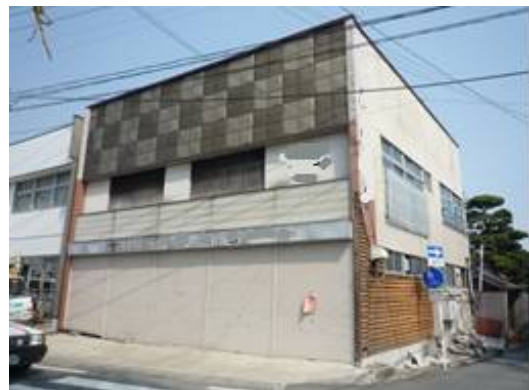
Photo 6.2-14 House with store with large story deformation
