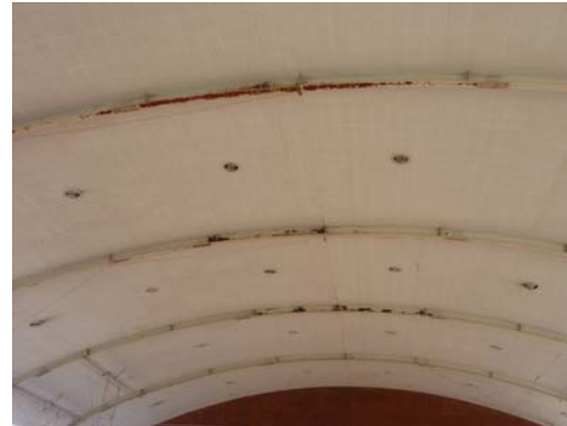
Photo 6.4-14 Peeling of paint of beams
