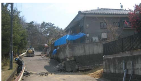
Photo 6.5-13 Damage to retaining wall and house by sliding and ground deformation
