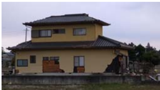
Photo 6.2-71 Falling down of mortar plastered wall
