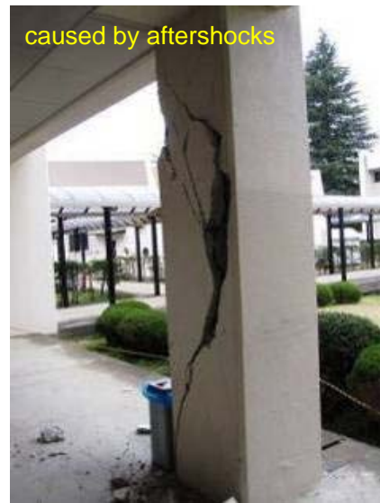
Photo 6.3-13 Shear cracks of first-story columns
