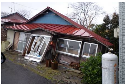
Photo 6.2-3 Damage of houses caused by ground transformation
