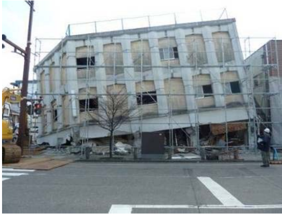
Photo 6.3-4 First-story collapsed building (Sukagawa city)
