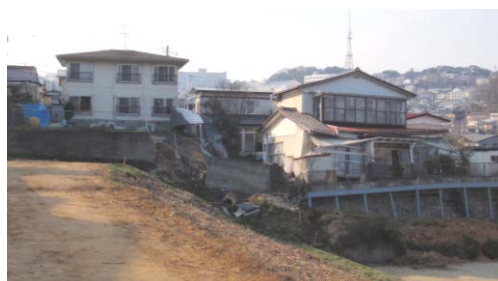
Photo 6.5-14 Group of houses damaged by sliding and ground deformation
