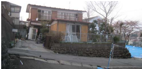
Photo 6.5-15 Damage to houses by sliding and ground deformation
