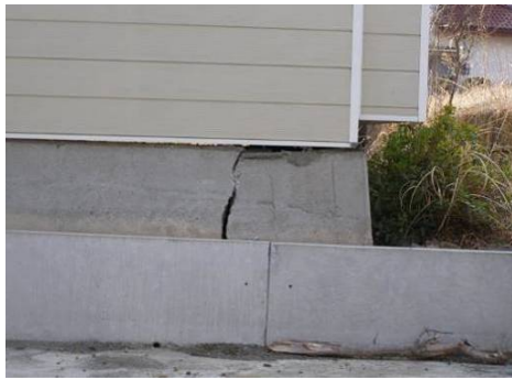
Photo 6.2-67 Crack of foundation
