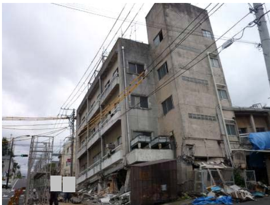
Photo 6.3-2 First-story collapsed building (Koriyama city)
