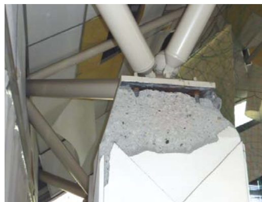
Photo 6.4-7 Spalling of concrete
