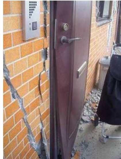
Photo 6.3-44 Damage of nonstructural wall and deformed door in same building shown in Photo 6.3-22
