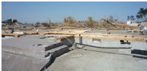
Photo.7.4-3. Foundations and sills remained.
