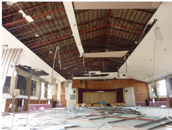
Photo 6.4-18 Dropping of extensive ceiling components
