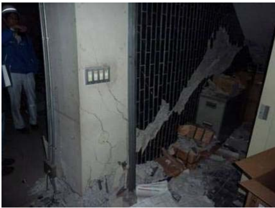
Photo 6.3-10 Shear crack on shear wall
