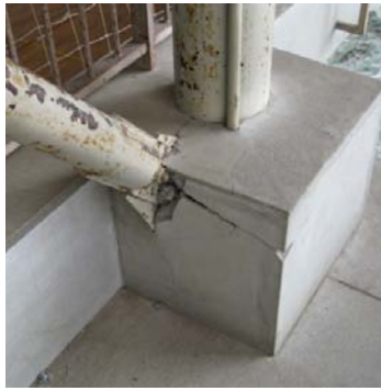
Photo 6.4-11 Cracking of column base concrete
