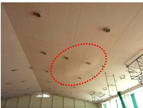
Photo 6.6-19 Sagging of metal furring suspended ceiling
