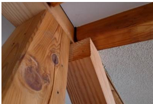
Photo 6.2-80 Slip of the wood brace
