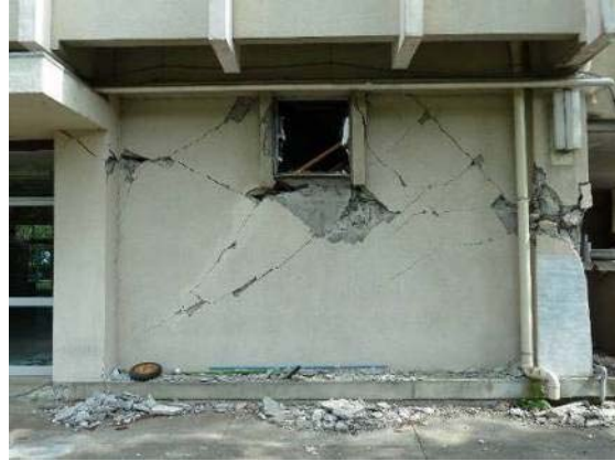
Photo 6.3-19 Shear failure of wall with opening
