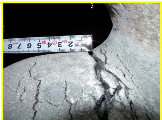
Photo 9.2-17 Lead damper and cracks on the surface
