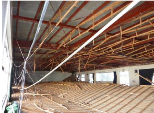
Photo 6.4-17 Dropping of extensive ceiling components
