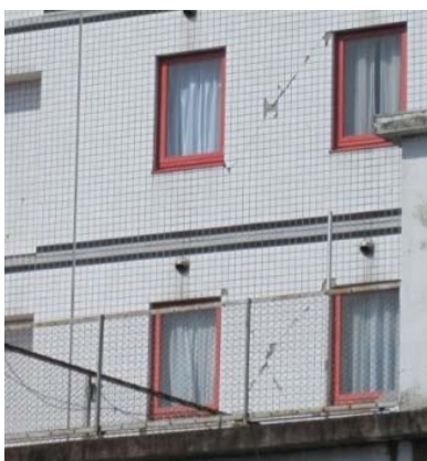
Photo 6.6-1 Detachment of ceramic wall tiles from damaged RC exterior wall
