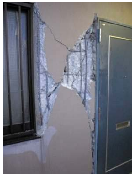
Photo 6.3-42 Shear failure of nonstructural wall
