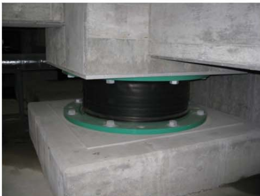
Photo 9.2-15 Natural rubber bearing
