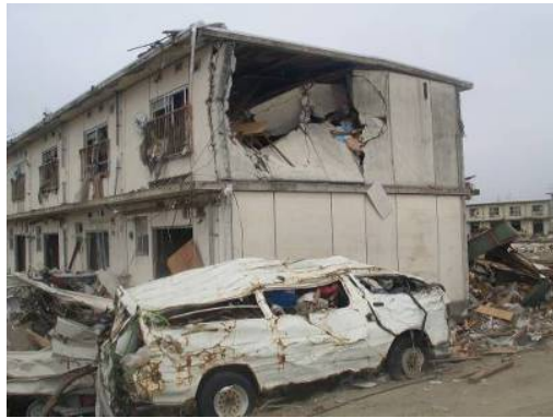
Photo 7.2-6 Wall opening generated by debris impact
