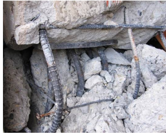
Photo 6.3-26 Close-up view of the bottom of SRC column
