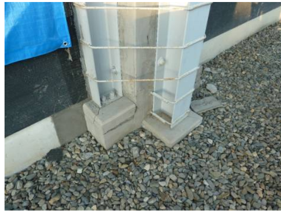
Photo 6.3-11 Column strengthened with H-shaped steel
