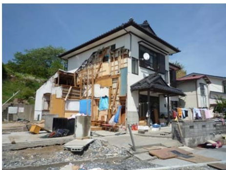
Photo 7.4-27. Wood house (1) remained under the flood water depth of over 7 m in Akasaki-cho, Oofunato city.
