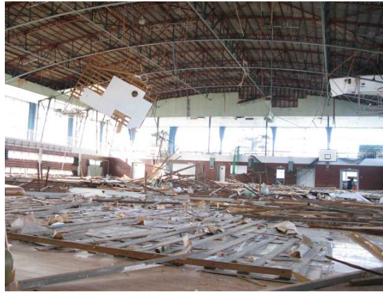
Photo 6.6-14 Falling of wooden suspended ceiling
