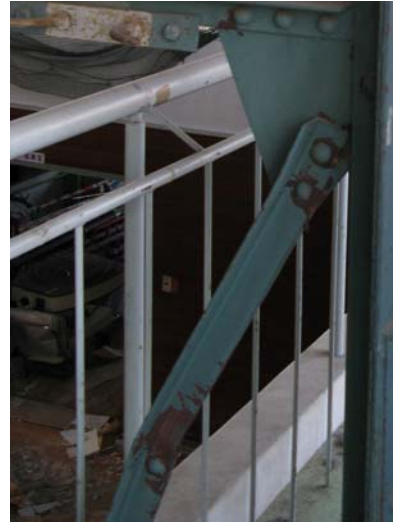
(b) Buckling of diagonal member
