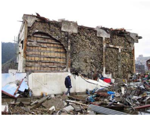
Photo 7.2-3 A 2-story reinforced concrete building that moved over the fence and overturned
