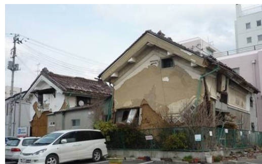
Photo 6.2-47 Failed warehouse with mud wall
