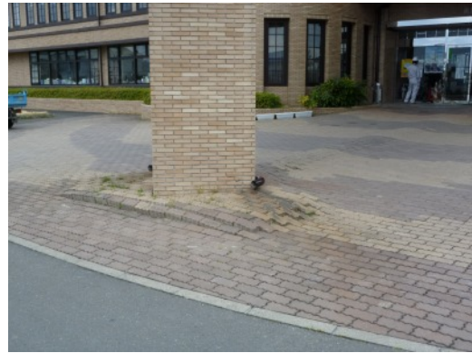
Photo 6.2-30 Ground deformation in Nango branch town office
