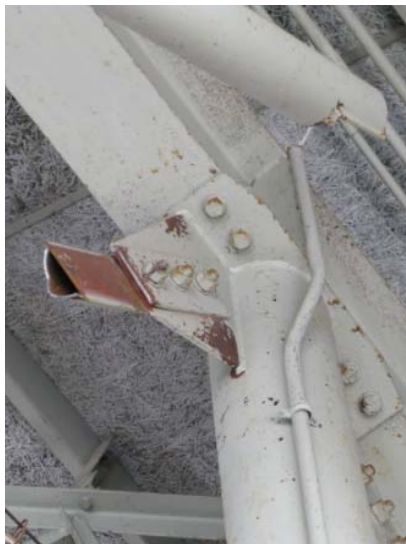
(a) Fracture at column top
