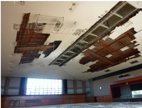
Photo 6.6-15 Falling of metal furring suspended ceiling
