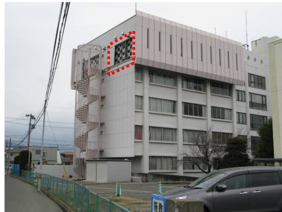
Photo 6.6-7 Detachment of AAC panels
