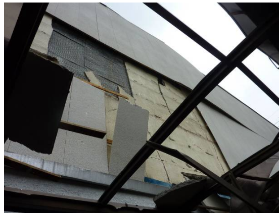
Photo 6.6-5 Damage to gymnasium gable end wall
