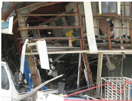
Photo 7.2-11 Tilted gabled roof frame
