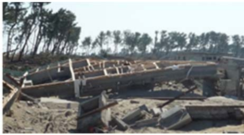
Photo.7.4-1. Foundations washed away.
