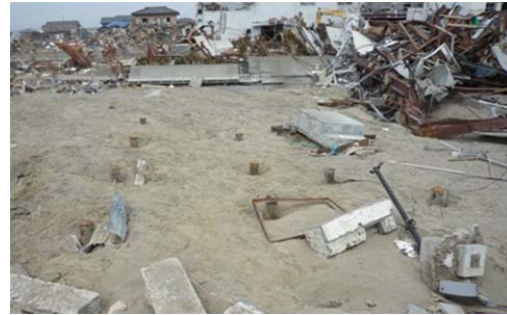
Photo 7.4-11. Steel tube pile left at the the original position ([2]) of photo 7.4-10.
