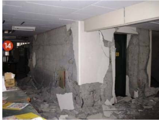
Photo 6.3-16 Failure of shear wall
