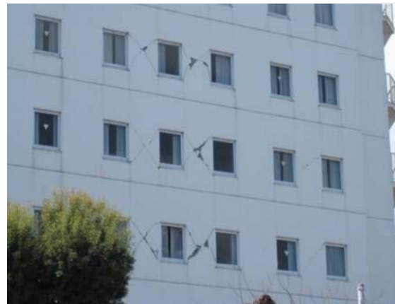
Photo 6.3-46 Shear crack on nonstructural wall
