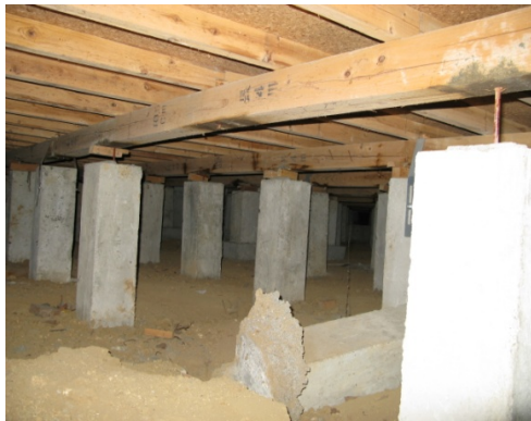
Photo 6.4-13 Overturning of floor strut
