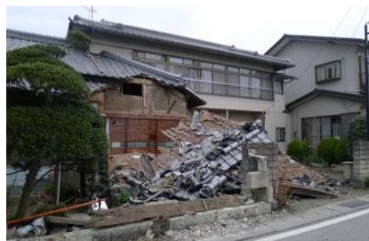
Photo 6.2-70 Breakage of entrance part.
