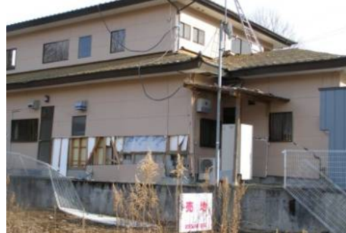
Photo 6.2-64 Damaged house due to deformation of residential land
