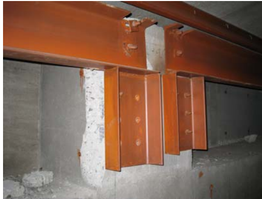
Photo 6.4-8 Pullout of hole-in anchors
