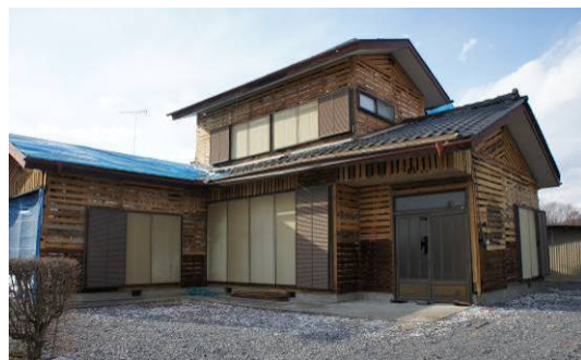
Photo 6.2-62 Damage of exterior mortar wall
