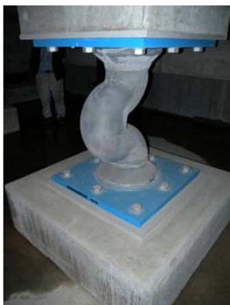
Photo 9.2-17 Lead damper and cracks on the surface
