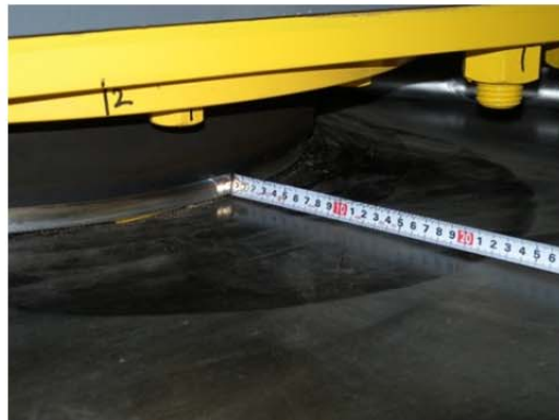
Photo 9.2-24 Trace of displacement of elastic sliding bearing
