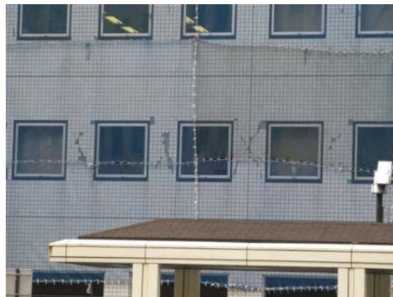
Photo 6.3-49 Damage of tile on exterior wall
