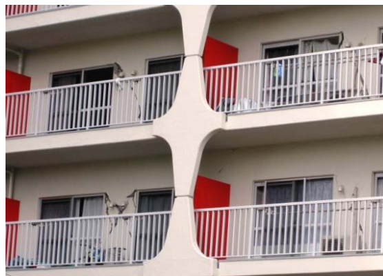
Photo 6.3-31 Shear cracks on mullion
