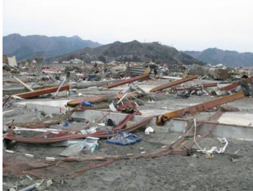
Photo 7.2-8 First-floor columns falling in the same direction
