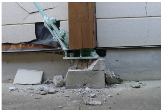
Photo 6.2-78 Breakage of the foundation concrete
