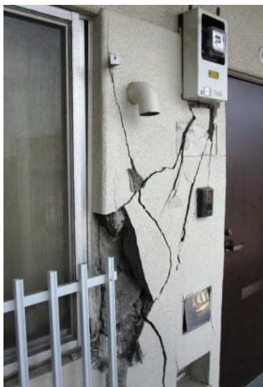
Photo 6.3-30 Shear cracks on nonstructural wall
