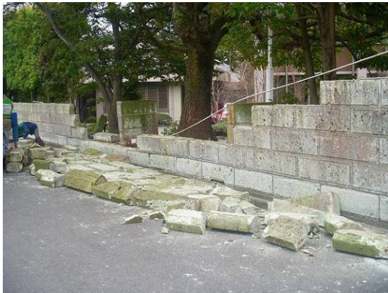
Photo 6.3-52 Collapse of stone masonry wall (Fukushima city)
