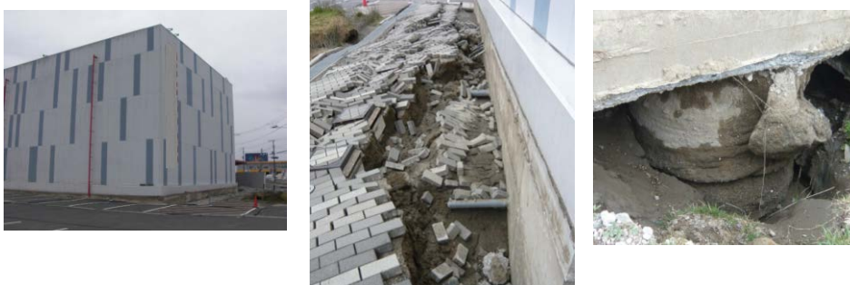
Photo 6.5-1 Situations around the commercial building and state of pile head
