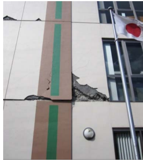
Photo 6.3-40 Separation of concrete of wing wall
