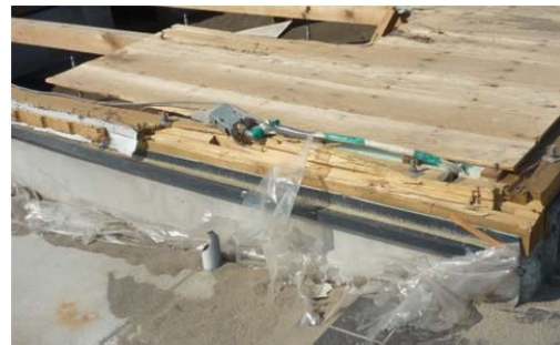
Photo.7.4-4. Sills, foundations and floor boards remained.
