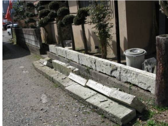
Photo 6.3-53 Collapse of stone masonry wall (Shirakawa city)
