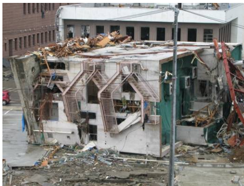
Photo 7.2-9 Overturning of a 3-story steel building
