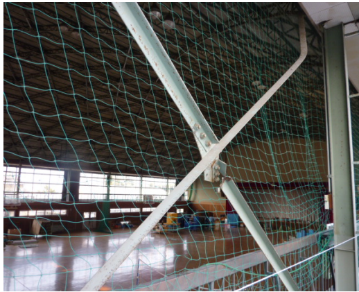
Photo 6.4-1 Buckling of brace
