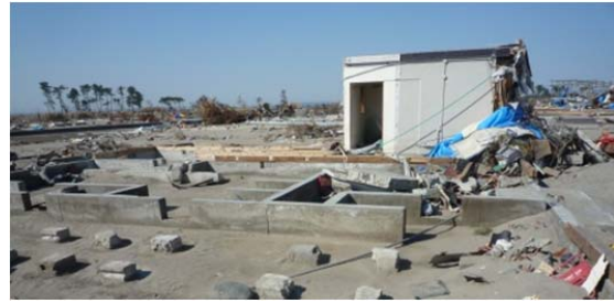
Photo.7.4-2. Only foundation remained.
