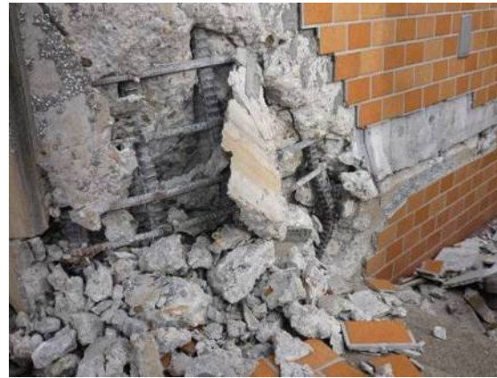
Photo 6.3-23 Damage at the bottom of SRC column
