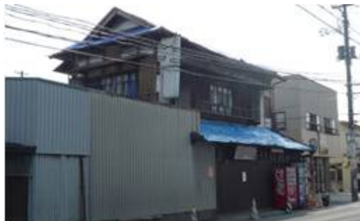
Photo 6.2-21 House with store with 2 nd story drift more than that of 1 st story
