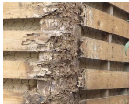
Photo 6.2-45 Deterioration and damage due to termite on column and wood lath of exterior mortar
