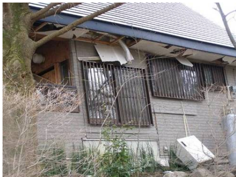
Photo 6.2-61 Failed ceiling of eave
