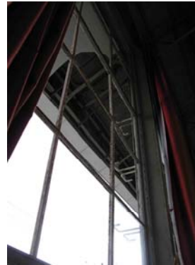
Photo 6.4-21 Falling of eave soffit
