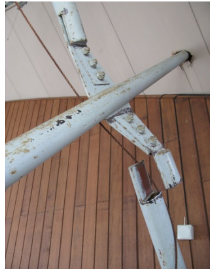
(b) Fracture at brace crossing
