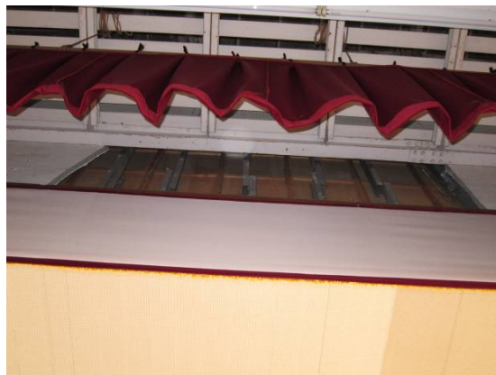
Photo 6.6-23 Falling of cement mortar finish above stage
