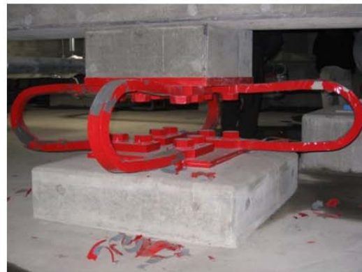
Photo 9.2-16 U-shaped steel damper
