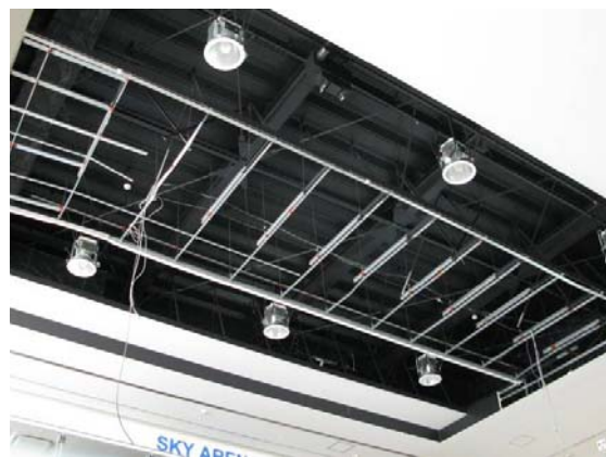
Photo 6.6-16 Falling of metal furring suspended ceiling
