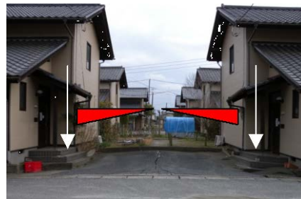
Photo 6.5-3 Subsidence of two houses enclosing vacant land
