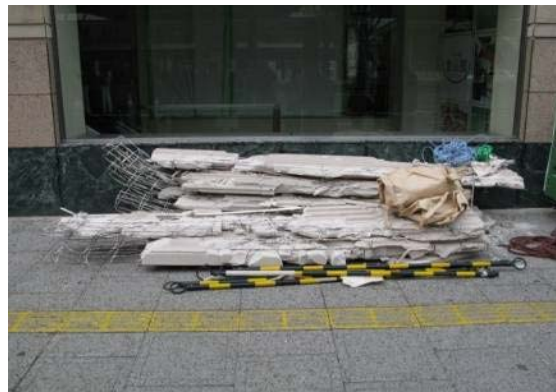
Photo 6.3-48 Dropped AAC panels
