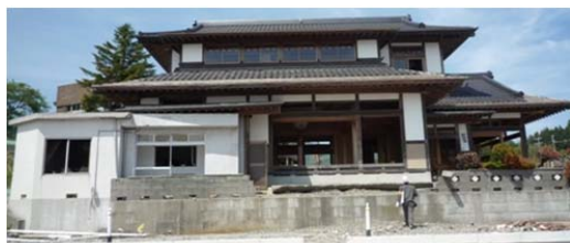
Photo 7.4-29. Japanese traditional wood house (5) which was not carried away under about 5 m flood water depth in Akasaki-cho, Oofunato city.
