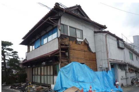
Photo 6.2-46 Collapsed stair hall
