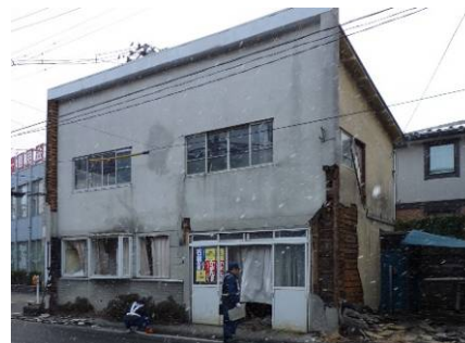
Photo 6.2-40 Drop off the mortar wall (Komatsujima)
