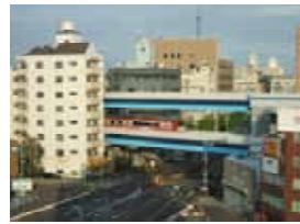
After elevated railway bridge
