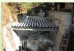
Debris flow breaker
