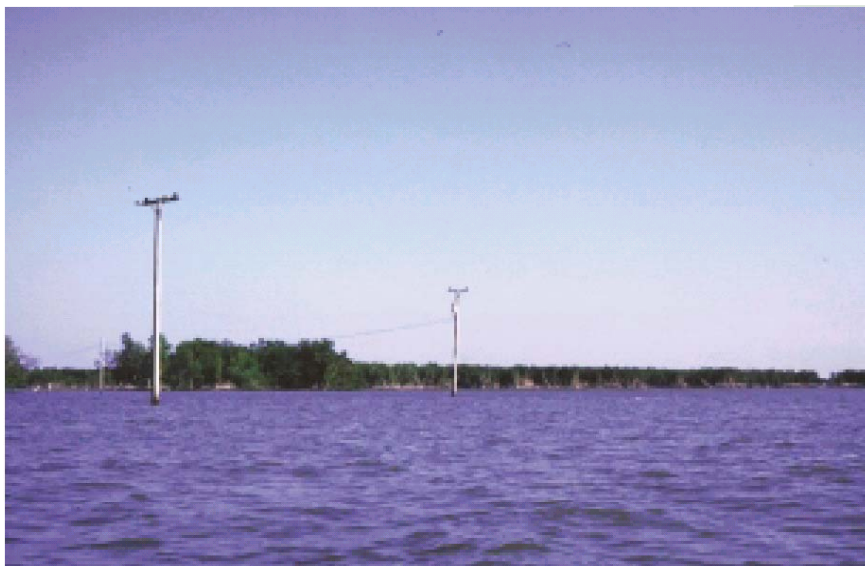
Erosion at the front
