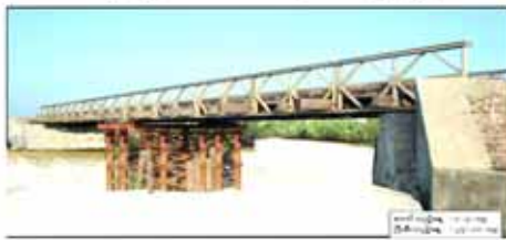
Pyew Cha Tawk Bridge ( 100 Feet )
