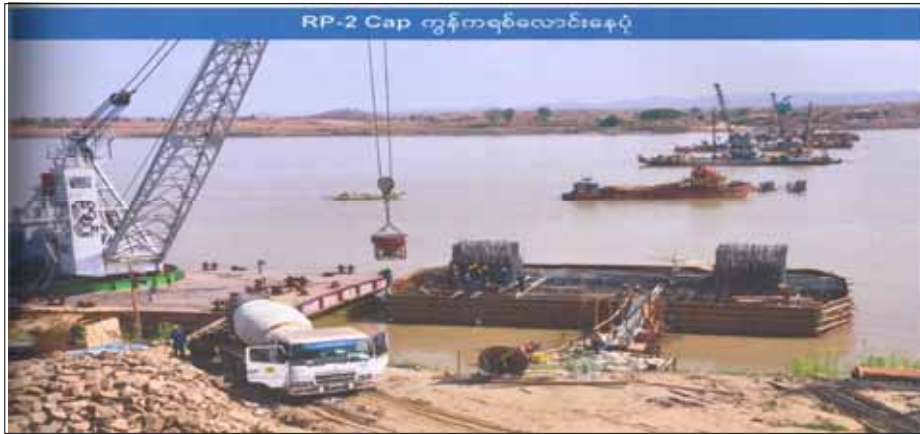
Ayeyarwaddy Bridge ( Malun)
