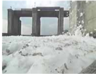
River surface covered with detergent foam from domestic effluent
