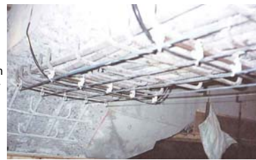
Titanium anode is set to re-bars
