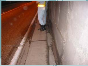
Deformed ditch in roadside
