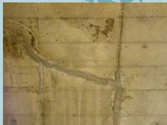
Crack/joint injection
