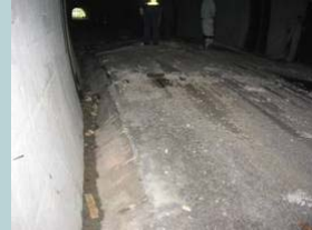
Heaving of road surface
