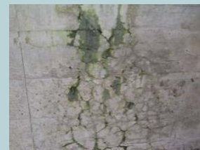
Alkali-aggregate reaction
