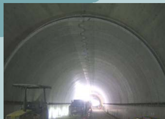
Internal reinforcement (Precast lining)
