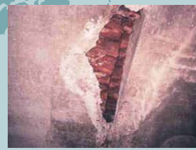
Shortage of concrete casting
