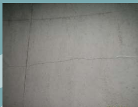
Shrinkage by temperature or moisture
