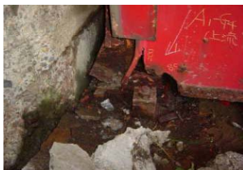
Broken girder edge caused by corrosion
