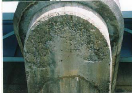
Honeycomb (bridge pier)
