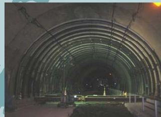
Internal reinforcement (Steel arch support)
