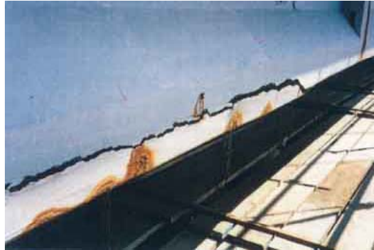
Chloride induced corrosion (PC girder) PC tendon was broken
