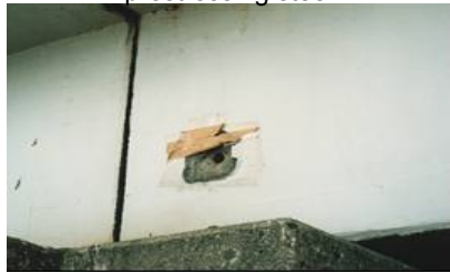
Corrosion and breaking of prestressing steel
