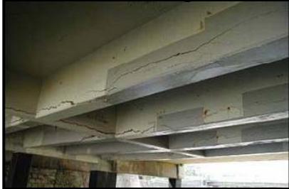
Corrosion and breaking of prestressing steel
