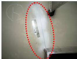
Crack occurred at the steel box girder
