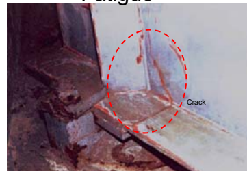
Crack by fatigue extending from lower flange to the web
