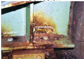
Local corrosion on girder edge
