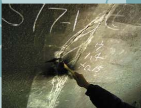
Crack by poor workmanship in setting form
