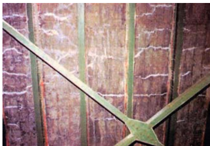
Transverse direction crack
