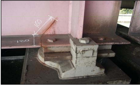
The crack progresses from sole plate of main girder to web
