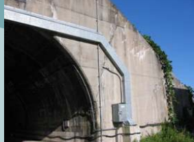
Crack on portal
