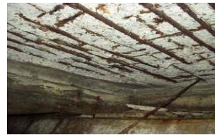
Rusting by Salt Damage
