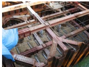
Anodes for steel pipe piles (Gray members)
