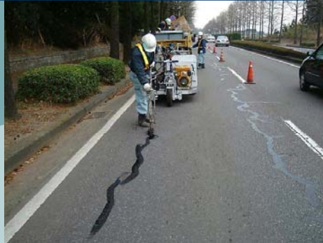
Preventative methods (ex. Crack Sealing)
