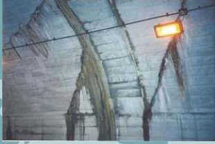
Crack on lining
