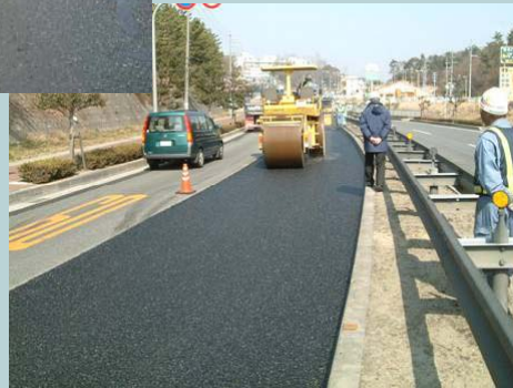
Repair methods (ex. Cut and Overlay)
