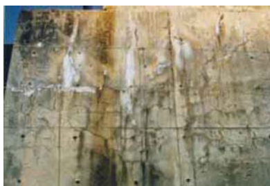
Alkali-Aggregate Reaction (Abutment)
