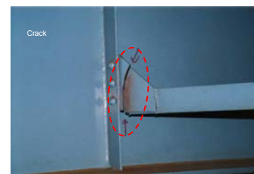
Crack by fatigue occurring in sway brace
