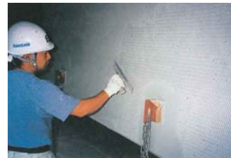
Applying adhesive on the sheets
