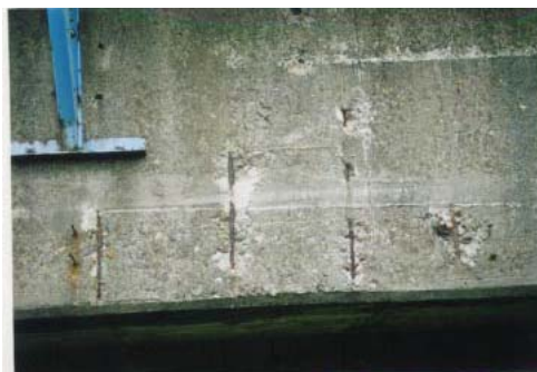
Shortage of cover concrete (bridge girder)
