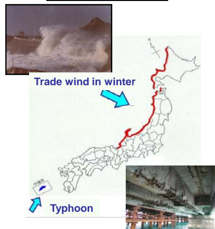
Damage of concrete by salt attack
