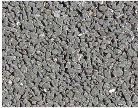
Drainage pavement (single-layer)
