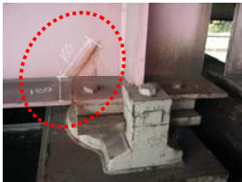
Crack occurred at the girder end
