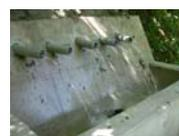
Horizontal gravity Drains
