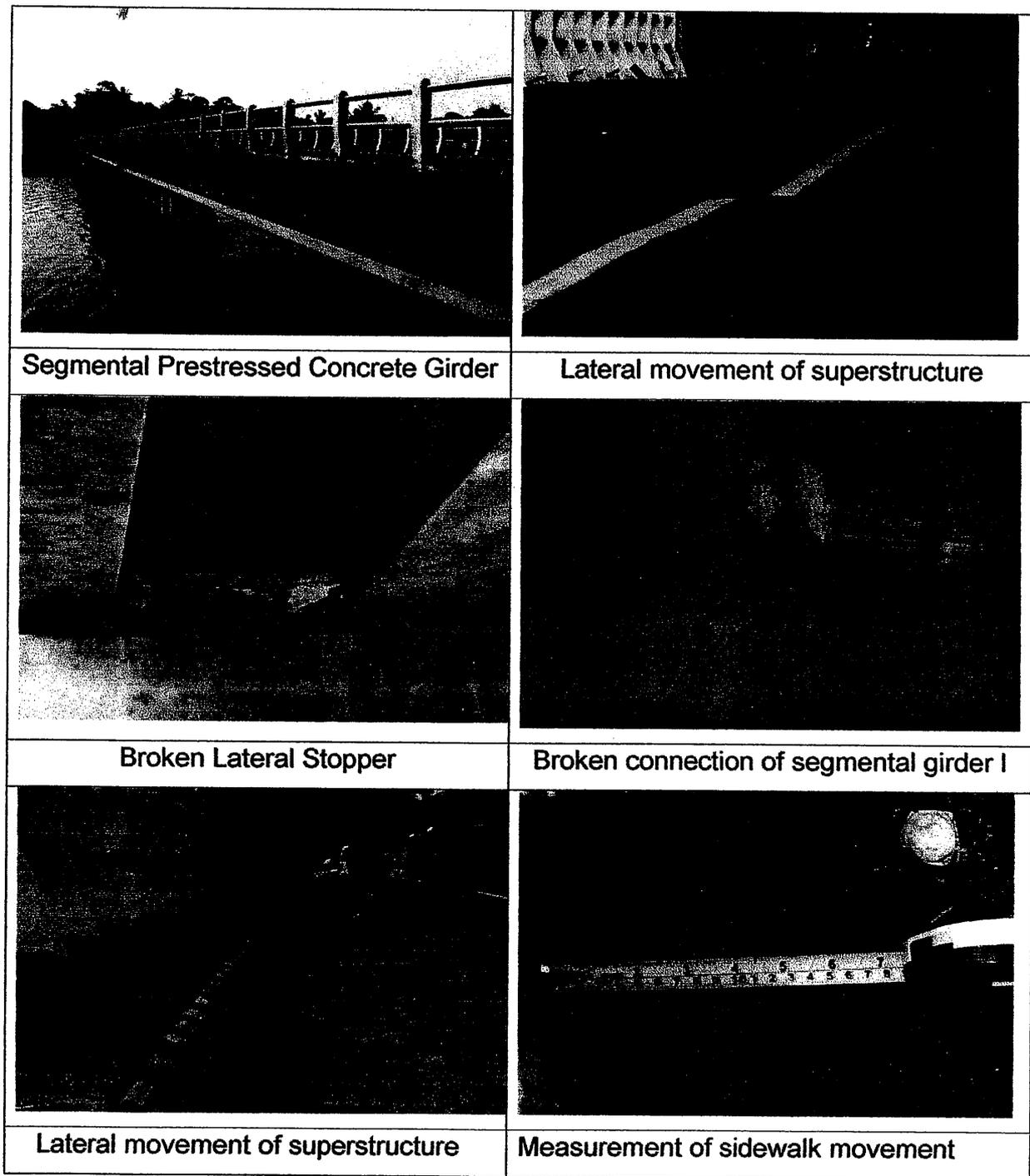
Figure 7. Damage of Lais Besar bridge
