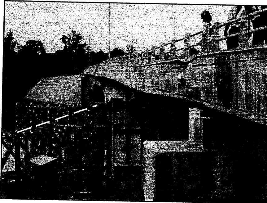
**Figure 3-2 Uneven bridge soffit in second loading test**
