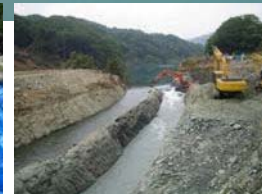
Work to expand channel completed July 5th
