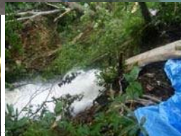
Forced drainage using drainage pump between June 19th and 22nd
