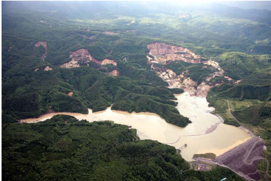
Downstream towards bottom, upstream towards top, of photo. Aratosawa Dam reservoir at center, with landslide occurring in its entire left upper tributary. The landslide has reached the reservoir. Multiple landslide areas apparent at left. Photo: Aero Asahi Corporation
