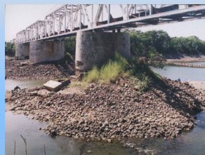
Exposed foundation (Cepiles Railway Bridge) Porong River
