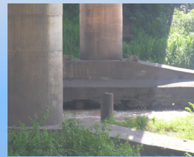
Scouring around Bridge Pier (Kademangan Bridge)
