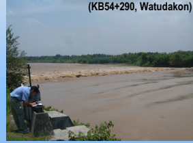
Degradation of riverbed in downstream section of Watudakon Siphon
