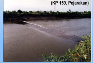
Degradation of riverbed and exposed conduit (old Bangil Tak Siphon)
