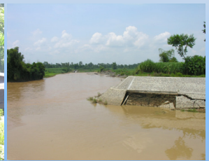
Damaged dike revetment (Right) (Ngrowo River and Brantas River Confluence)
