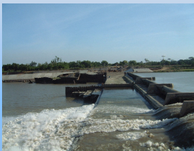
Damaged Jatimlerek Rubber Dam Brantas River
