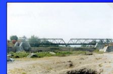
Sabo dam in Putih river, Mt. Kelud area (East Java) to prevent degradation of riverbed.
