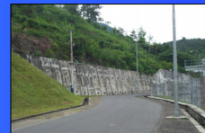
Anchor method to prevent slope failure implemented in West Sumatera.
