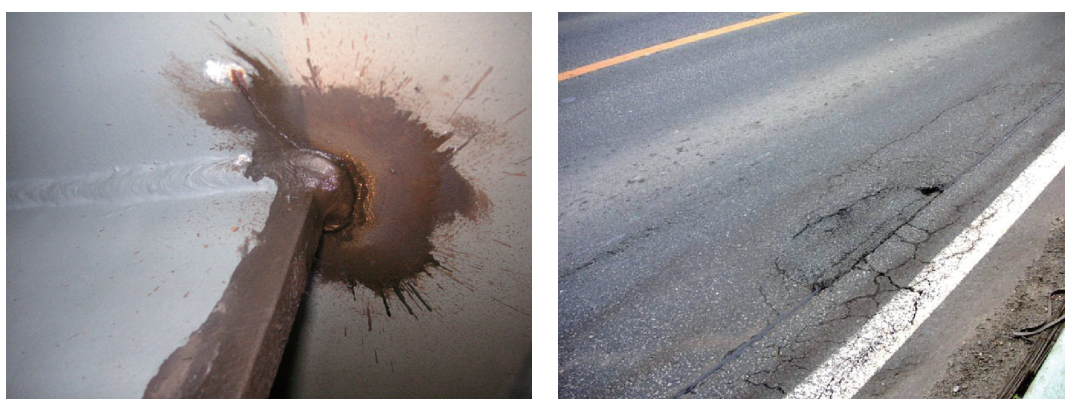
a) 鋼床版の疲労き裂
