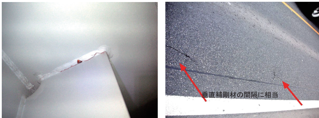
a) 鋼床版の疲労き裂
