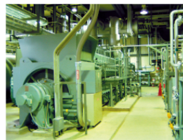
Gas Engine + Generator
