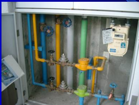
Example of distinction by color-coding the pipes (Yellow is reclaimed wastewater, blue is drinking water)
