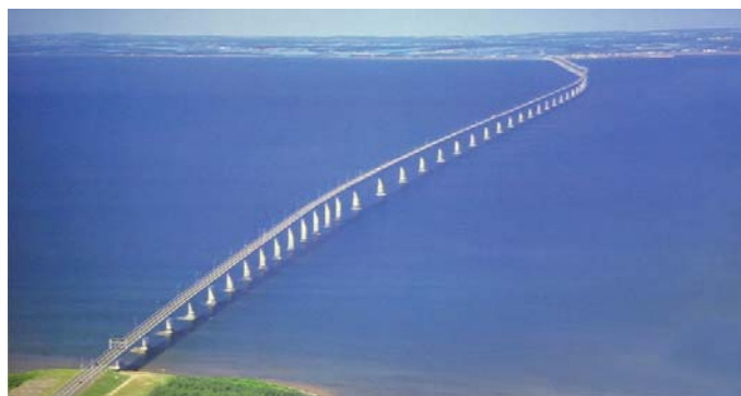
Fig. 2.2 Confederation Bridge in Canada. Completed in May 1997. Length 12.9km, 60 m high navigation span (including 1 m allowance for sea-level rise).
