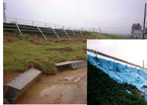
Slope collapse has occurred due to insufficient infiltration safety
