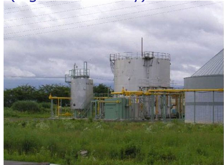
Gas storage tank by adsorption (e.g. Tsuruoka city)
