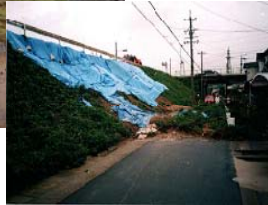
Slope collapse has occurred due to insufficient infiltration safety
