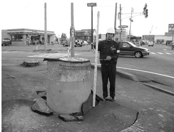
Photo1. A lift-uped manhole in Niigata-ken Chuetsu Earthquake
