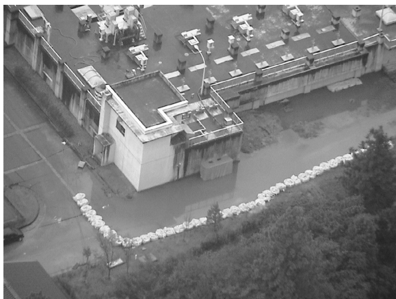
Photo2. A temporary settlement pond and a disinfection plant in Horinouchi Treatment Plant
