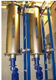
Dynamic ultrafiltration units (2 x 7,4 m 2 ) and pressure station for care-water distribution
