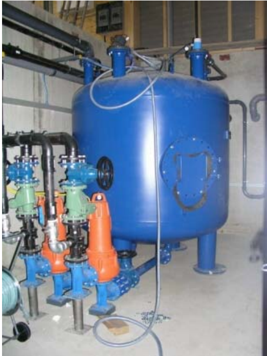
Vacuum station installed in the water house
