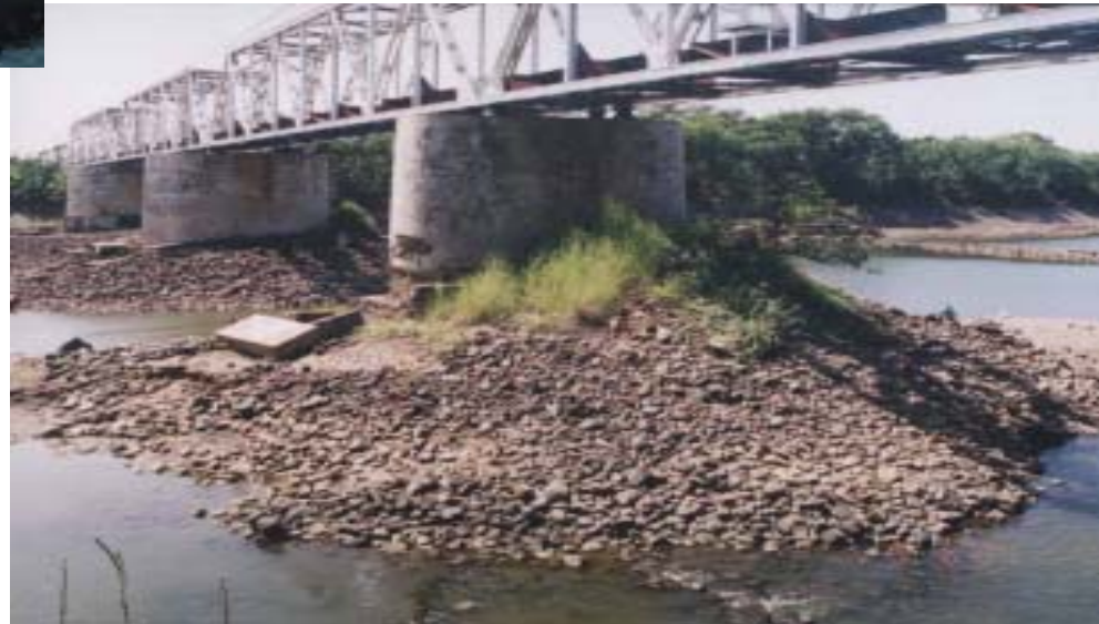
Exposed foundation (Cepiples railway bridge), Porong River
