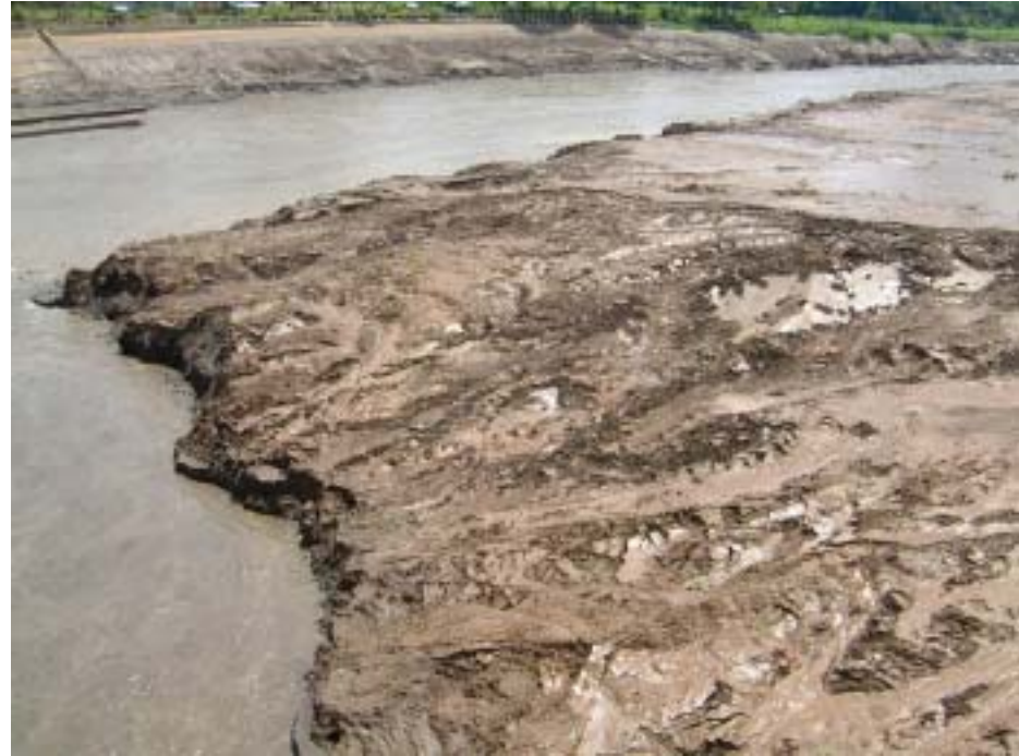
Sediment on left bank (on high water channel)
