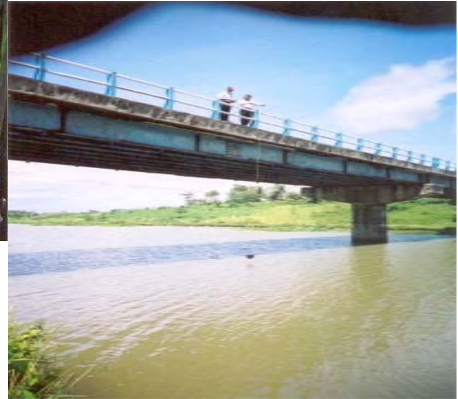
River water sampling point, bridge location
