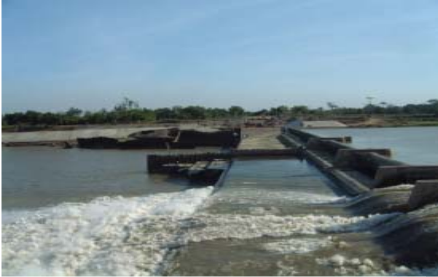
Damaged Jatimlerek Rubber Dam, Brantas River
