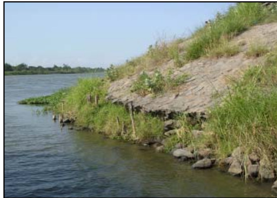
Damaged dike revetment (Right) KB 85, KB 86 (Megaluh)
