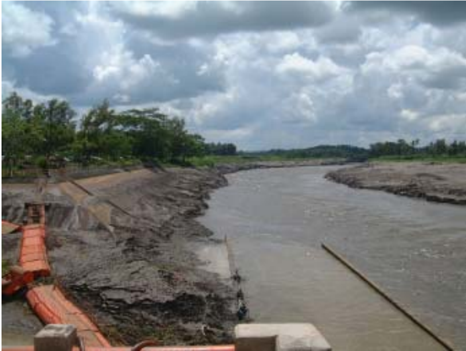
Sediment around upstream section of power intake
