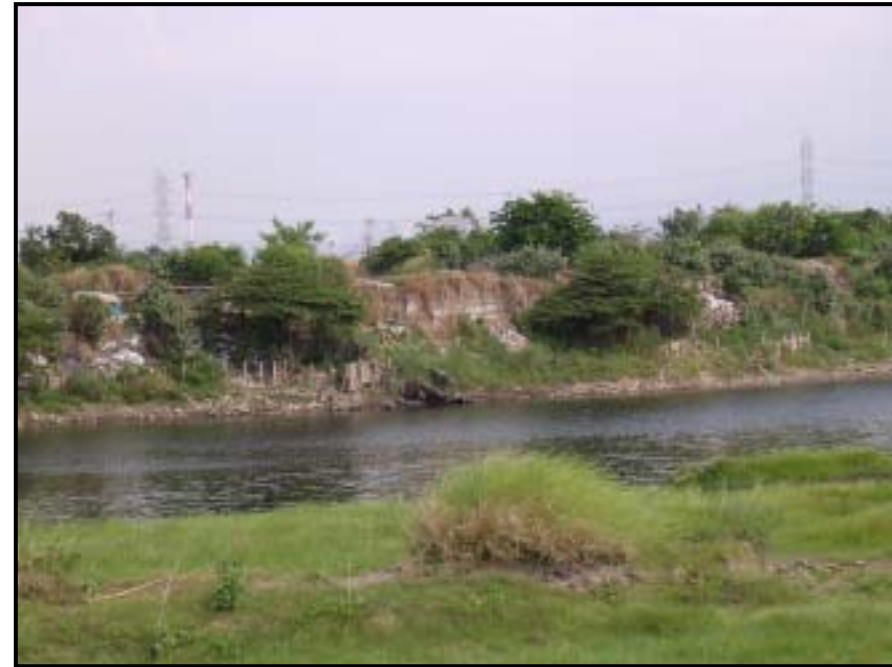
Collapsed revetment and dike (Right)
