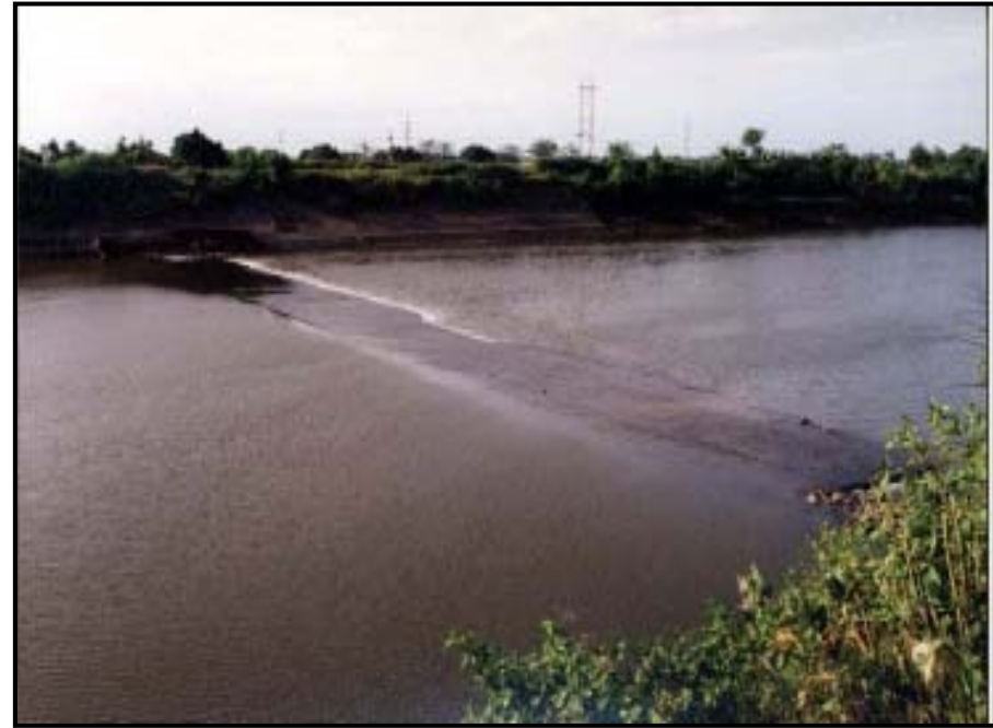
Degradation of riverbed and exposed conduit (old Bangil Taak Siphon)
