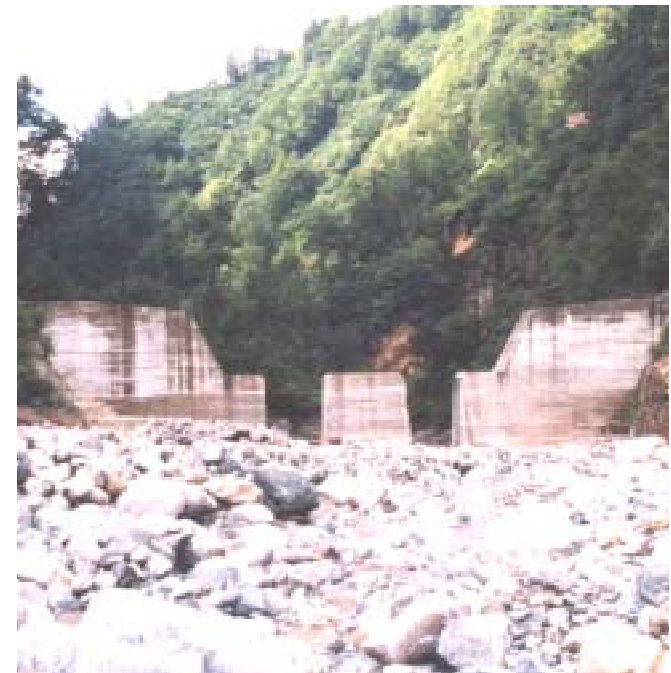
Example of concrete slit dam
