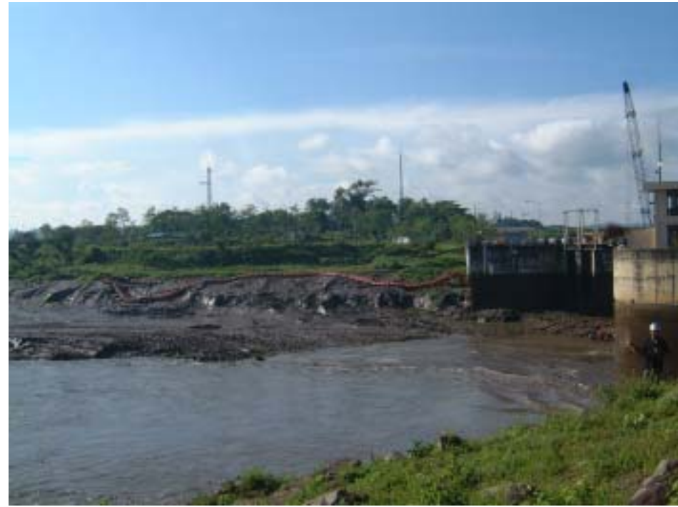
Sediment around power and irrigation intakes
