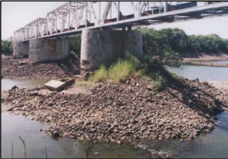
Exposed Foundation (Cepiples Railway Bridge)
