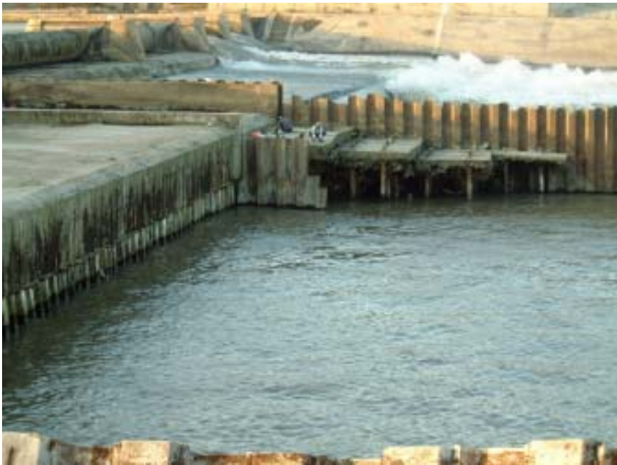
Damaged Jatimlerek Rubber Dam
