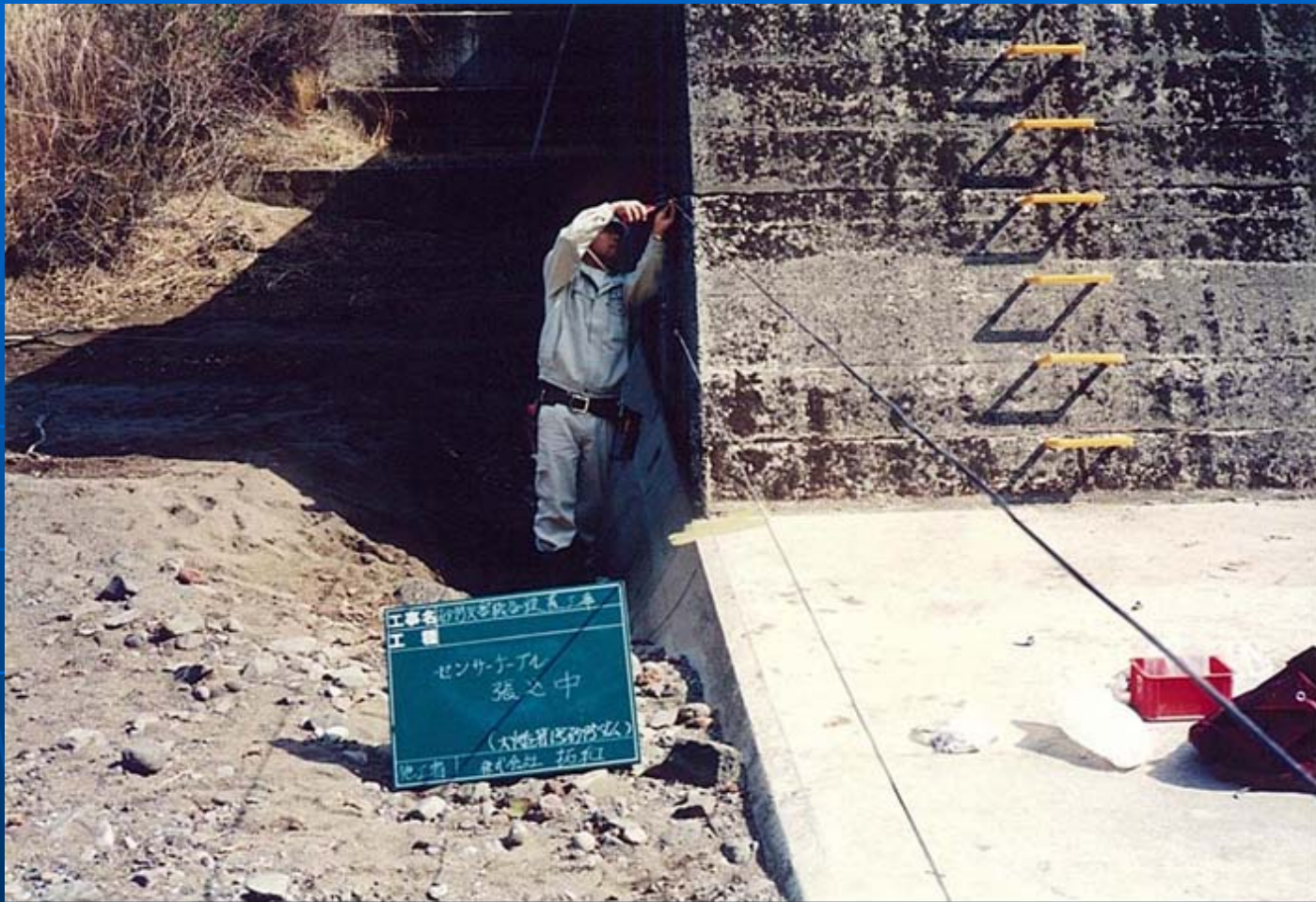
Sensor Being Installed
