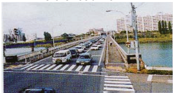
Before road work
