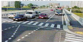
After road work
