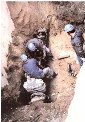
Repairing work of distribution main pipe
