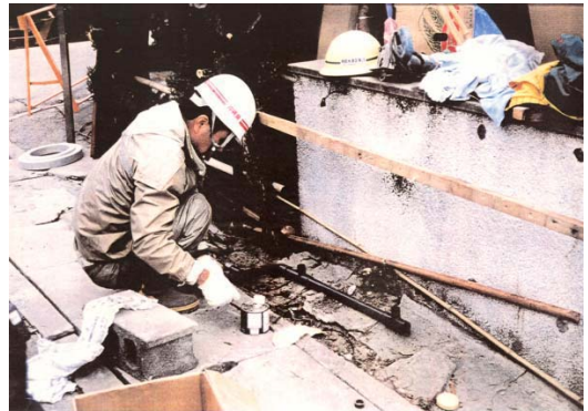
Repairing of service pipe
