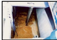
The inside of a aeration tank
