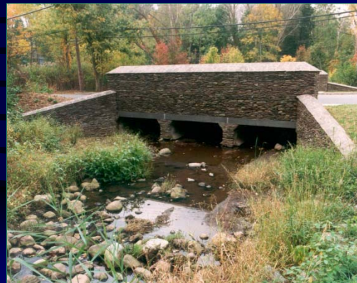
View of stone-faced headwall and forebay.
