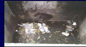
Catch Basin Without Hood 0% Retention
