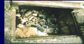
Catch Basin With Hood 50%-85% Retention
