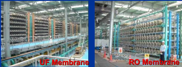
A Plant Under Construction in FUKUOKA 50,000m 3 /day
