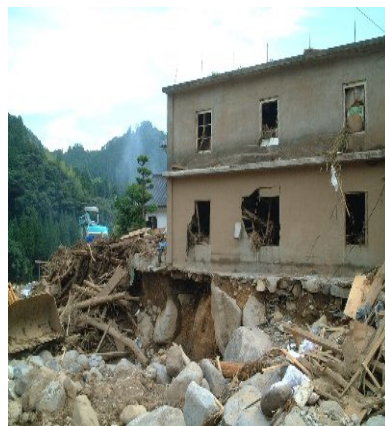
Photo.5 The debris flow that struck the Hogawachi community
