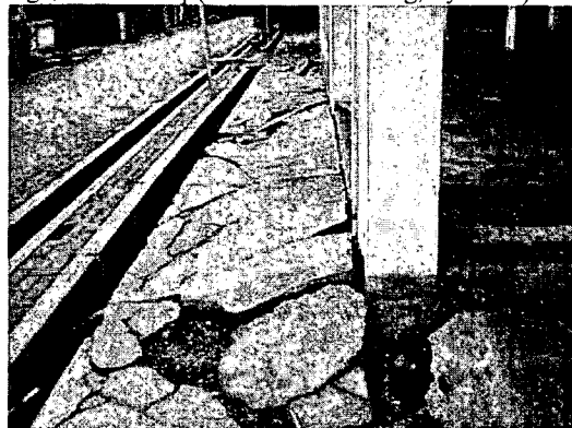
Photo 4.6~7. Example of flat house, Bandarhardjo, north Semarang, completed in 1998. subsidence in 4 years is observed at its foundation
