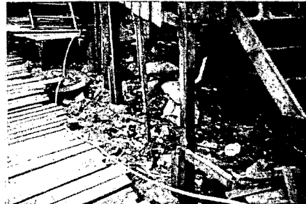
Photo. 2.7.7. Condition of underneath of house which is full of garbage
