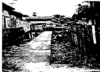
Photo 2.6.2: Wooden footpaths made of ulin timber
