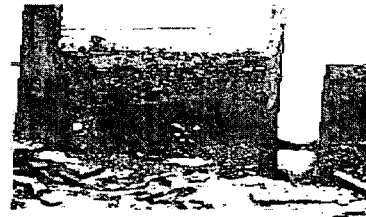
Photo 2.6.6 and 2.6.7: Bottom beam is decayed because of the quality of wood
