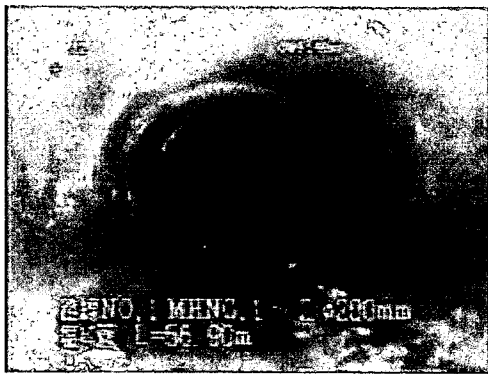
Photo 1 (before installation, July, 1999)
