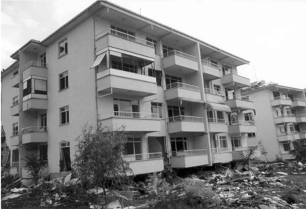
Photo 1 RC Building in Gölçüç which pancaked during the 1999 Koçaeli earthquake.
