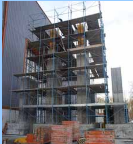
Construction of the large-scale bridge piers outside of the ELSA Laboratory
