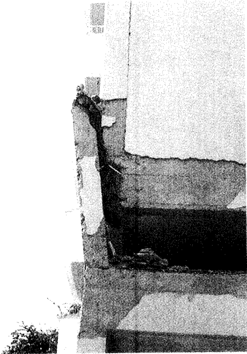
1) Visible settlement and/or inclination of floor
