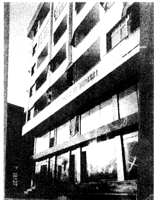
4) Rank C: Diagonal cracks observed in upper stories. Keeping out is needed near the building.
