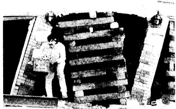
(2) Shoring with double crossed wooden layers
