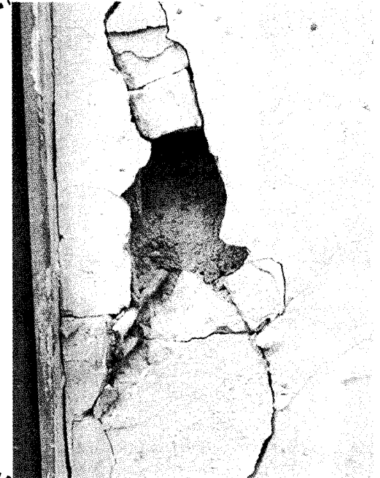
3) Big crack is observed on mortar. But take the mortar away, no crack is observed on the face of concrete.
