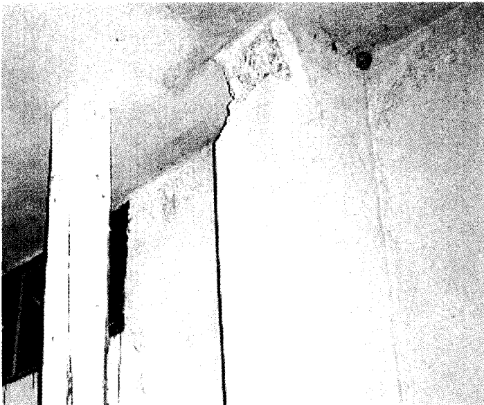
7) Big shear crack and spalling of cover concrete is observed at the top of column.
