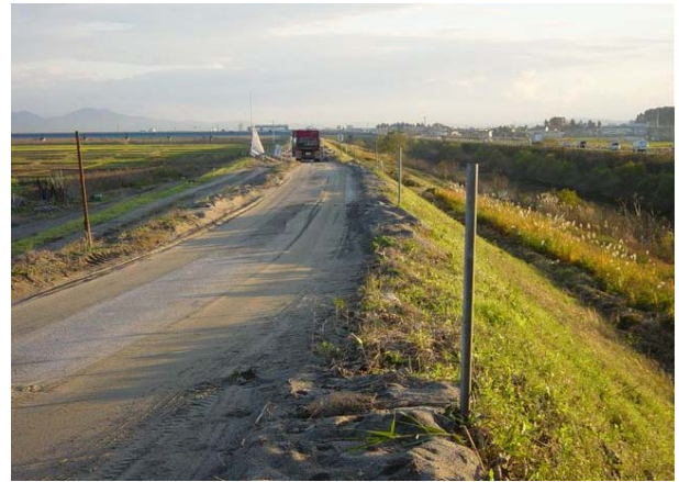
(a)のり肩を残し堤防天端が陥没
