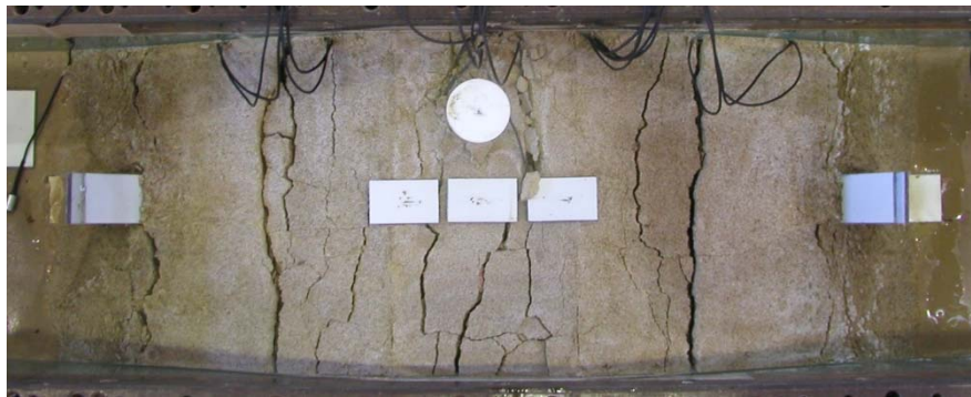
天端沈下0.75m
