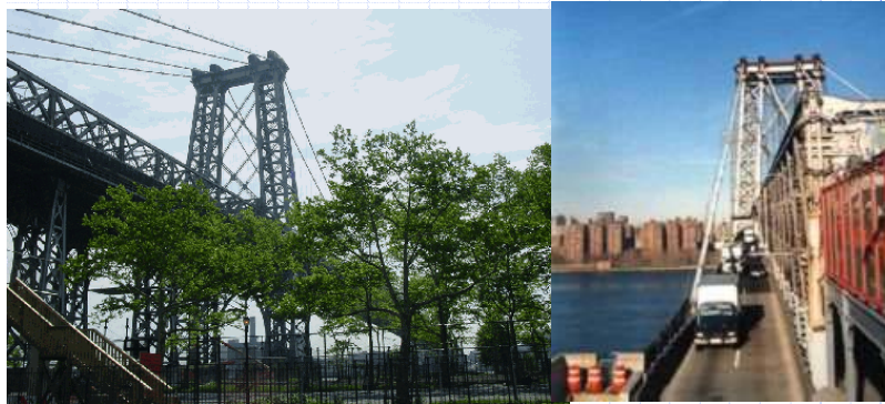
Williamsburg Bridge Open on December 19, 1903 (110 years)
