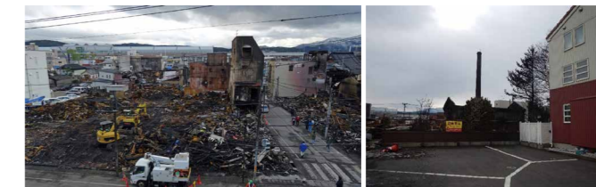
Photo 1. Damage in the center of the fire damaged district
