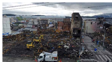
Photo 1. Damage in the center of the fire damaged district
