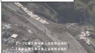
View of damage (road subsidence)
