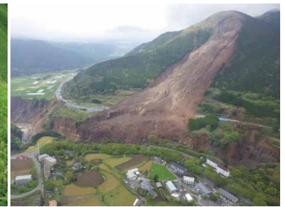
Photo 2. Large-scale collapsed slope near Aso Bridge
