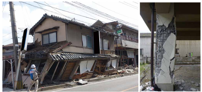
Photo State of damage to buildings (left: wooden, right: RC)
