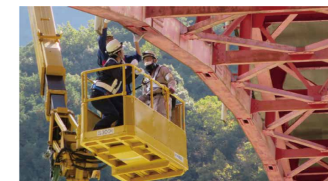
View of Diagnosis of Sarukai Bridge
