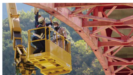
View of Diagnosis of Sarukai Bridge
