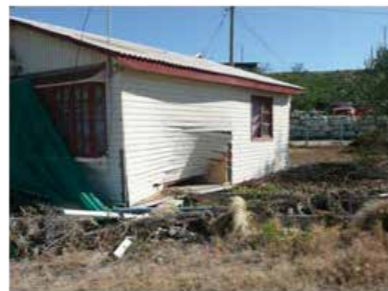
Photo : damaged house (in Puerto Aldea)
