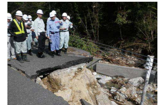
Photo: Masayuki Yabu, Head of the Pavement and Earthworks Division, giving technical guidance concerning the restoration of a collapsed road (Nikko City)
