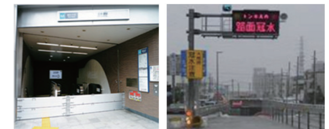
Photos: Inundation Countermeasures (left: installing a waterproof plate, right: road submersion information)
