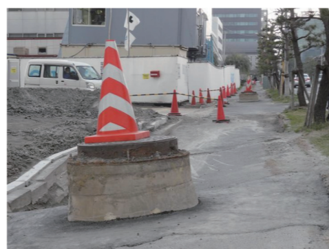
Photo: Manhole pushed up by Liquefaction
