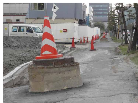
Photo: Manhole pushed up by Liquefaction
