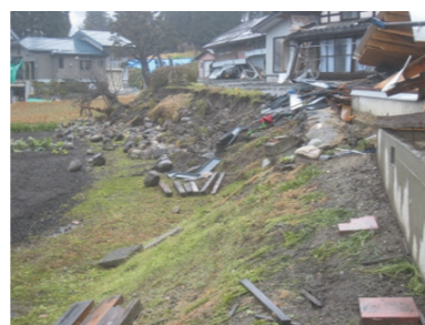
Photo: Collapsed Stone Wall
