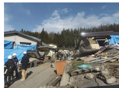
Photo: Collapsed House
