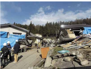
Photo: Collapsed House
