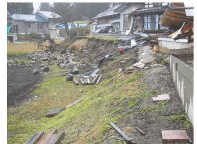
Photo: Collapsed Stone Wall
