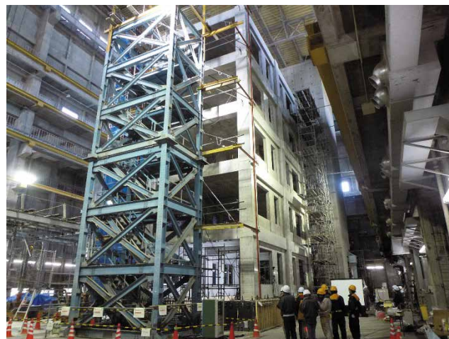
Photo: Loading test of a Full-scale Five-story Building
