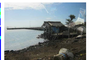
Photo: Damages in Estancia Port
