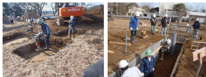
Performing the experiment Laying the PVC pipes
