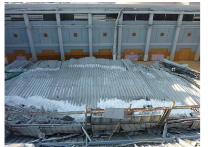
Photo: Collapsed roof of a gymnasium
