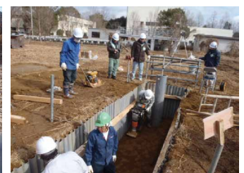
Laying the PVC pipes
