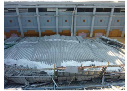
Photo: Collapsed roof of a gymnasium
