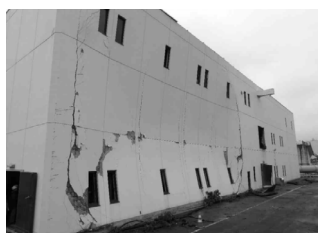
Building damaged by a tsunami
