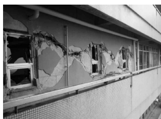
Damaged non-structural wall
