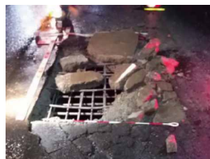
Example of the collapse of RC deck slabs
