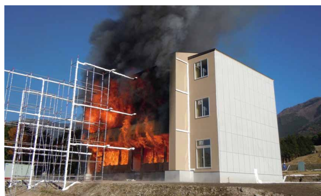
View of the building 137 minutes after ignition, when the fire had spread to the 1st and 2nd stores
