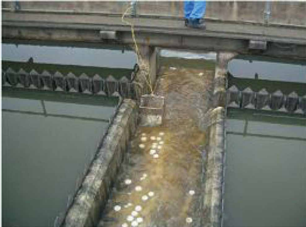
State of disinfection by solid chlorine at the early emergency restoration stage
