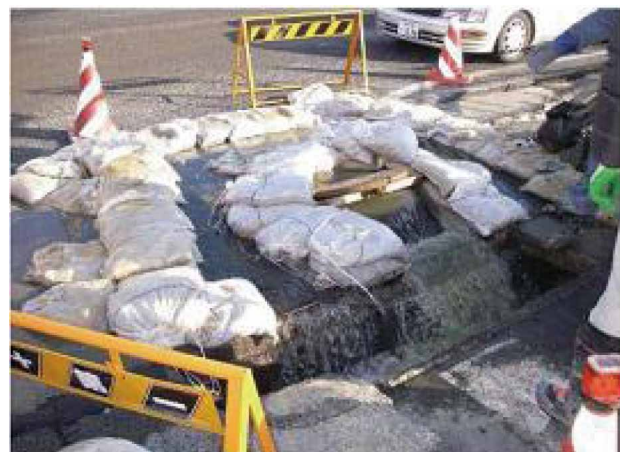
Example of the use of sandbags to guide sewage to a nearby channel
