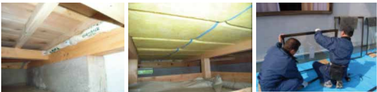
Examples of energy conservation renovation methods (from left, blocking air flow in walls, adding insulation below the floor, sash window attachment method)
