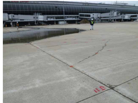
Cracks and puddles on an apron
