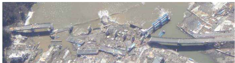
Bridge with Part of its Spans of its Superstructure Washed Away (Photo provided by the Tohoku Regional Development Bureau)
