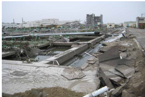
View of Damage at the Minami Gamo Wastewater Treatment Center (Sendai City)
