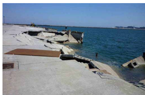
Collapsed Quaywall (Soma Port)
